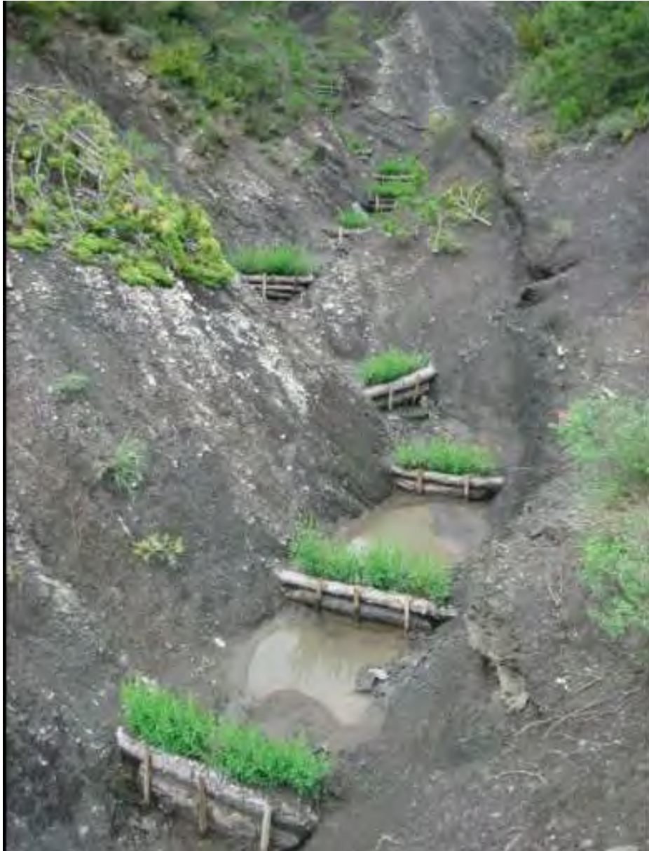
Figure 17. Bioengineering structures aiming at trapping sediment in France (F. Rey 2018).
