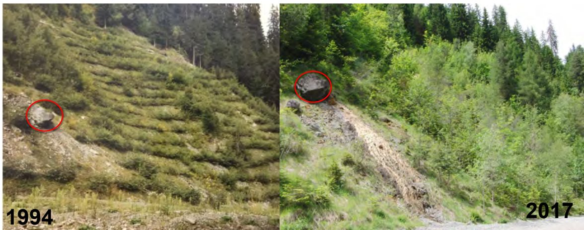
Figure 15. Documented development of a bioengineering measure (edge layers, analogous to spaced-planted trees) in the Swiss alps, showing the transition from classical bioengineering setup in 1994 to a protection forest stand (modified from Schwarz 2017).
