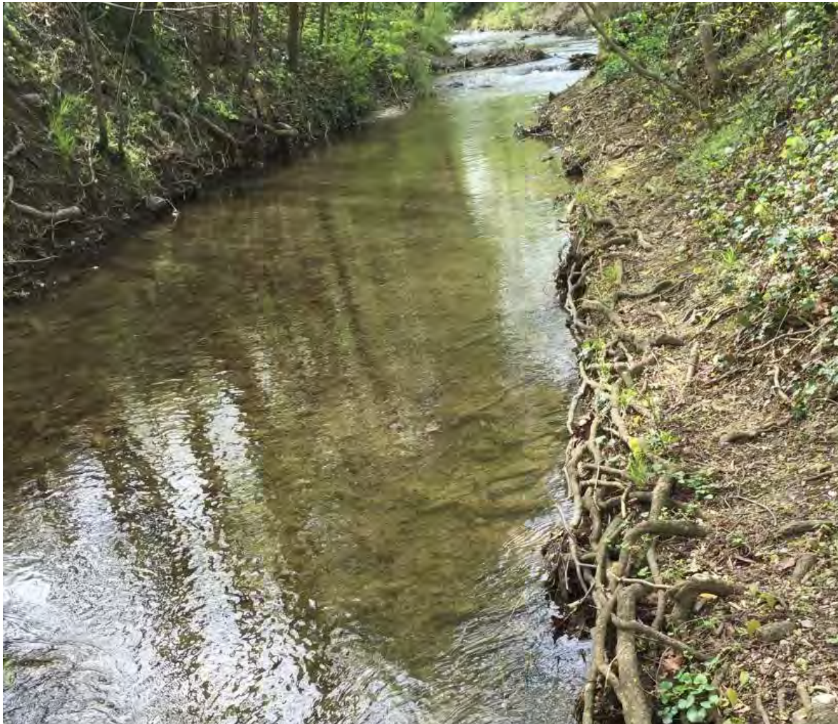
Figure 18. Example of conditions in which roots along a stream bank may contribute to reduce the magnitude of hydraulic erosion processes (source M. Schwarz).
