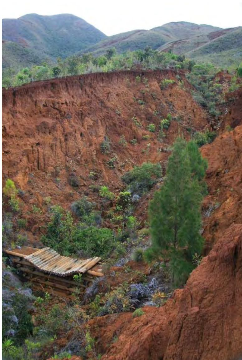
Figure 16. Gully channel stabilization with wooden dams mixed with vegetation in New Caledonia (F. Rey 2018).
